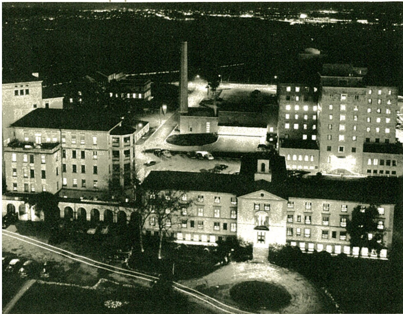
Seen at night from atop the Professional Building are the Clinic Building, left; the nursing residence and U. of H. College of Nursing, foreground; the new hospital building, right, and the Arabia Shrine Clinic, left background.
